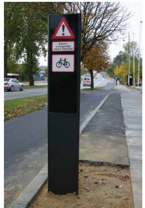
The sign lights a warning to cyclists that they risk meeting a right turning lorry in the signalized intersection ahead.
