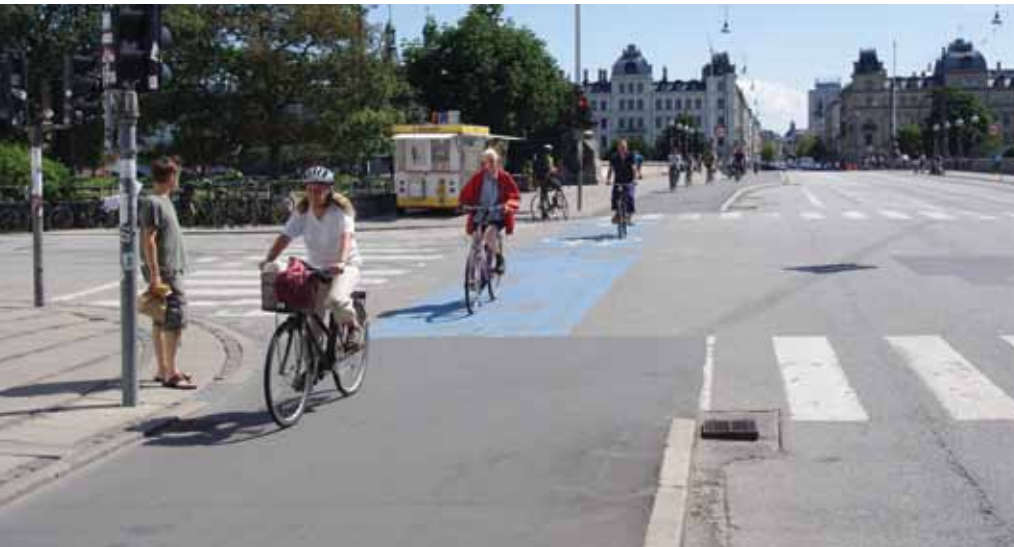
Cycle track capacity issues can be addressed by widened cycle tracks on the sections of the network where there isn't enough room. The blue cycle crossing shows the former cycle track width. Dr. Louises Bridge, Copenhagen.
