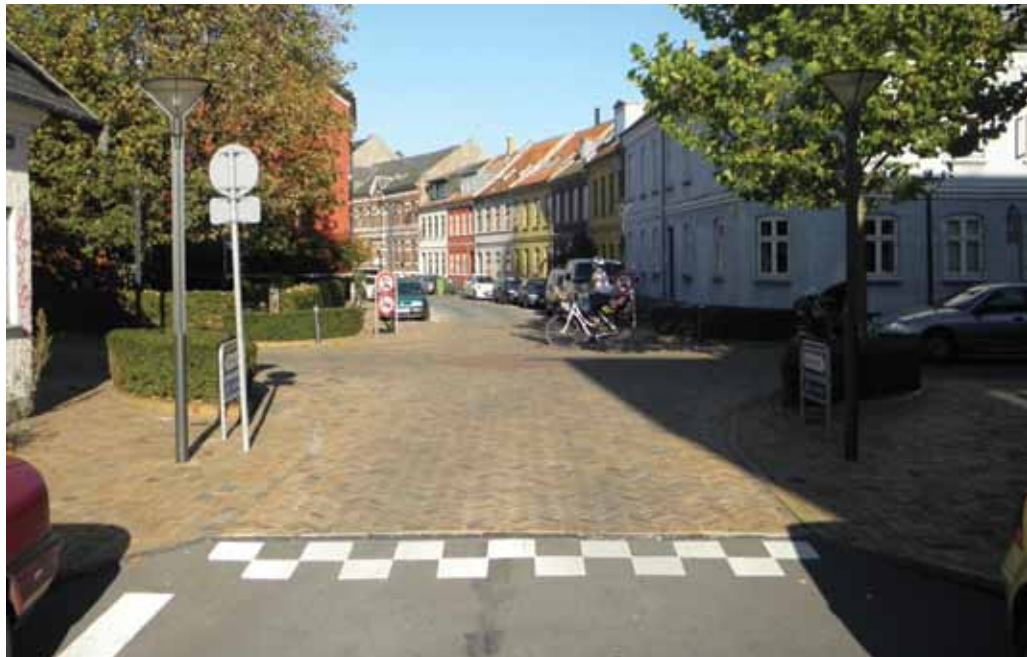
The crossing is raised to pavement level.
