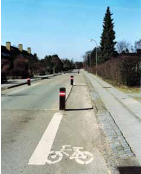
The road sweeping vehicle does not necessarily sweep around bollards.
