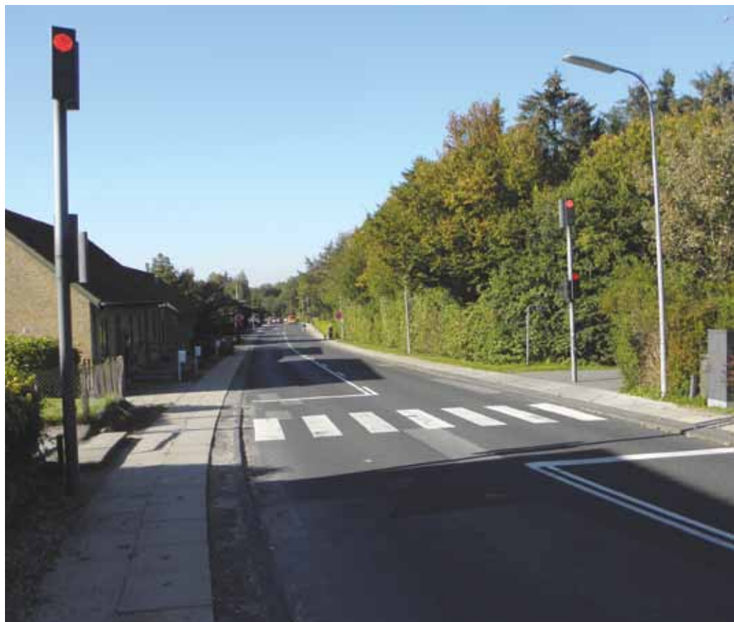
The traffic signal is activated by detectors on the path so cyclists rarely have to stop for other crossing road users.
