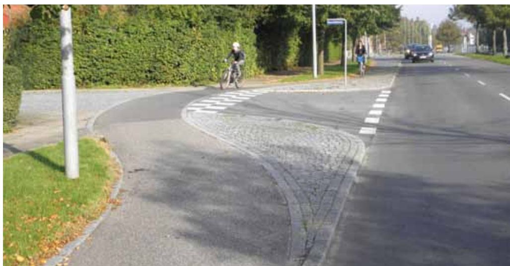
Set-back cycle track. The bend means that cyclists can't bike through the intersection faster than 20 km/h; motor vehicles have a waiting area on the outer edge of the cycle track.
