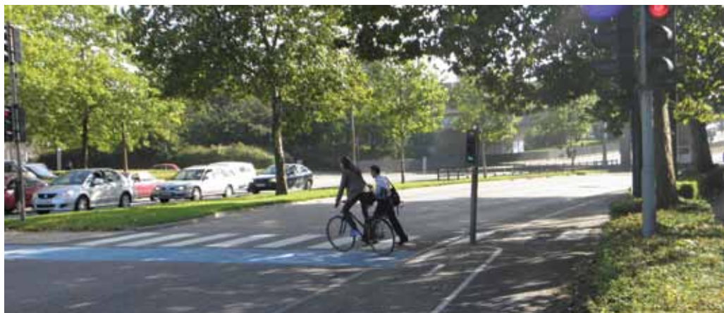
Blue cycle crossing at signalized intersection where there are major streams of oncoming, left turning motor traffic.
