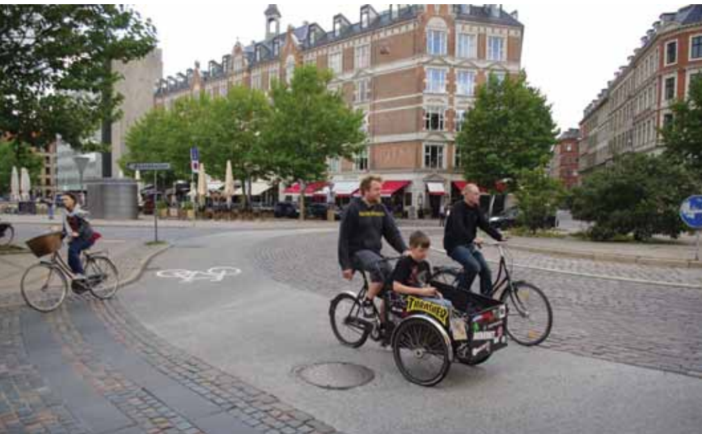
Traffic calmed roundabout with tarmacked cycle lane all the way around. Halmtorvet, Copenhagen.
