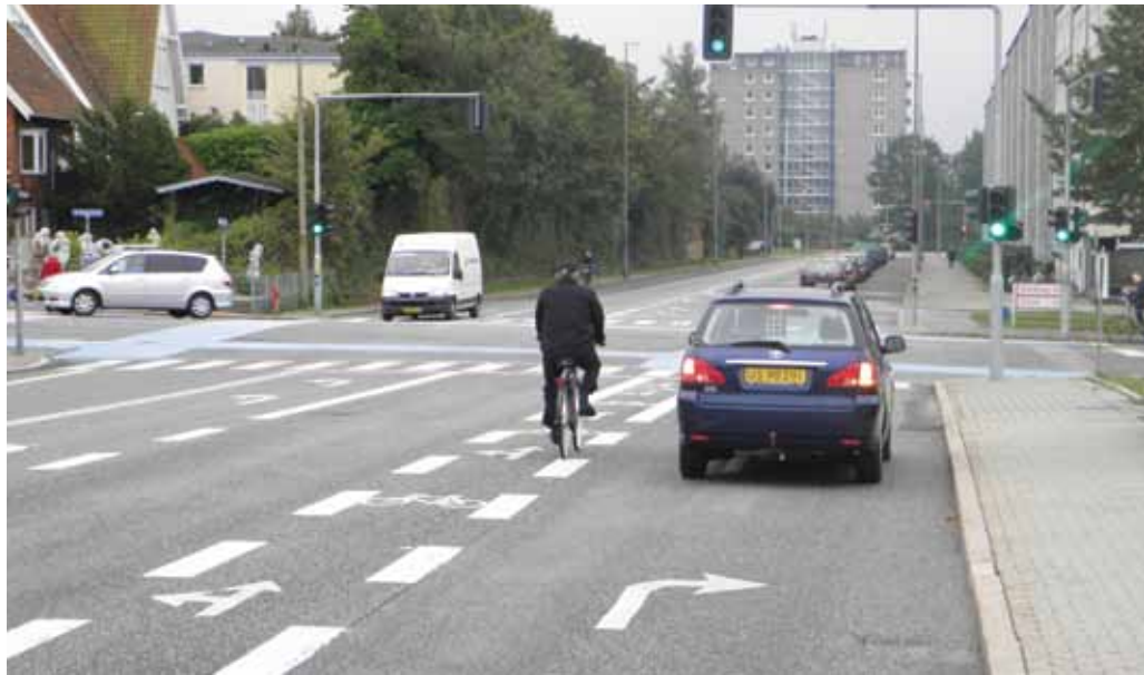
Cycle crossing between motor vehicles' right turn lane and lane for straight ahead traffic.
