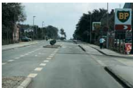
Small curve radii may encourage turning motorists to reduce speed when the cycle track is not continued across the side road.
