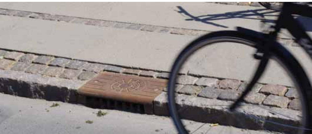
When cycle tracks are very narrow, rain water gullies built into the kerb remove rough spots making the cycle track more bikeable.
