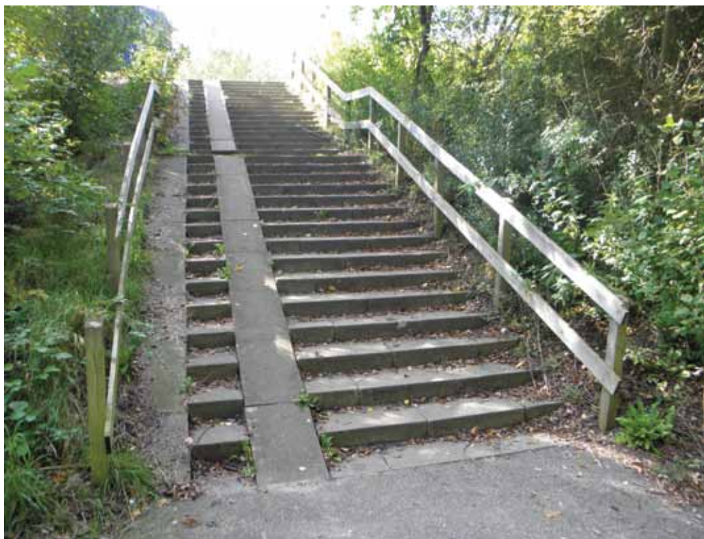
Combined bike and pram ramp.
