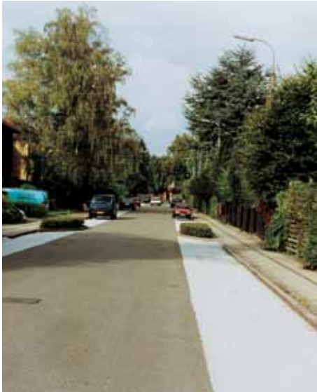
Parking lanes prevent slomling.
