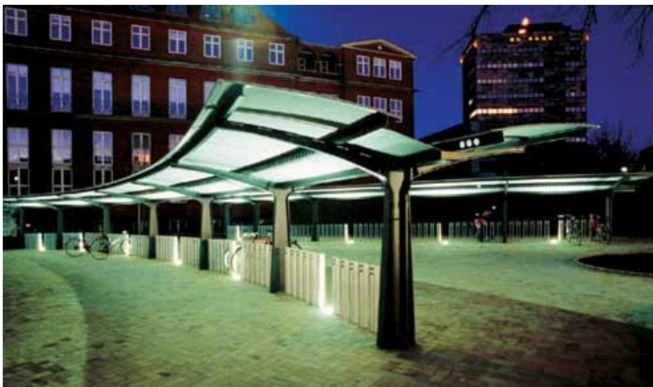
Covered bicycle parking facility at Kinopladsen, Odense, at night.
