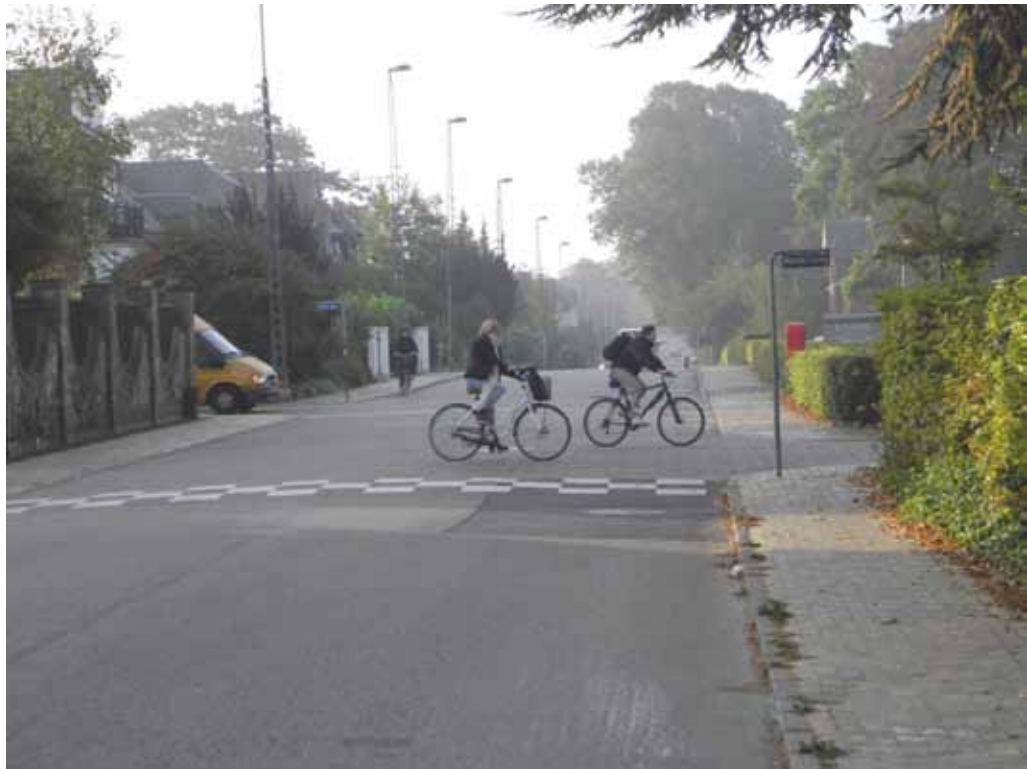
Speed humps are a particularly effective traffic calming measure. The hump can be installed over the entire width of the road without a cycle gap, which in this case is best for cyclists and cheaper to install.
