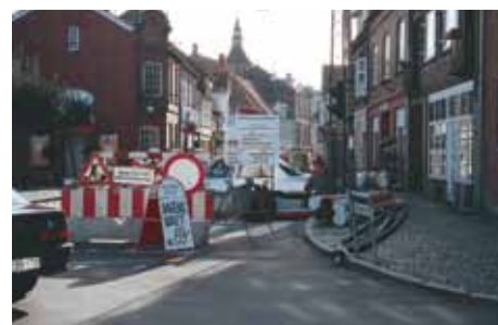
One way of improving cycling facilities is during utility construction.
