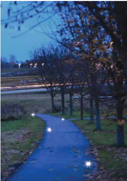
When there is no street lighting solar powered LEDs can be an excellent means of indicating the course of the path, here outside Aarhus.
