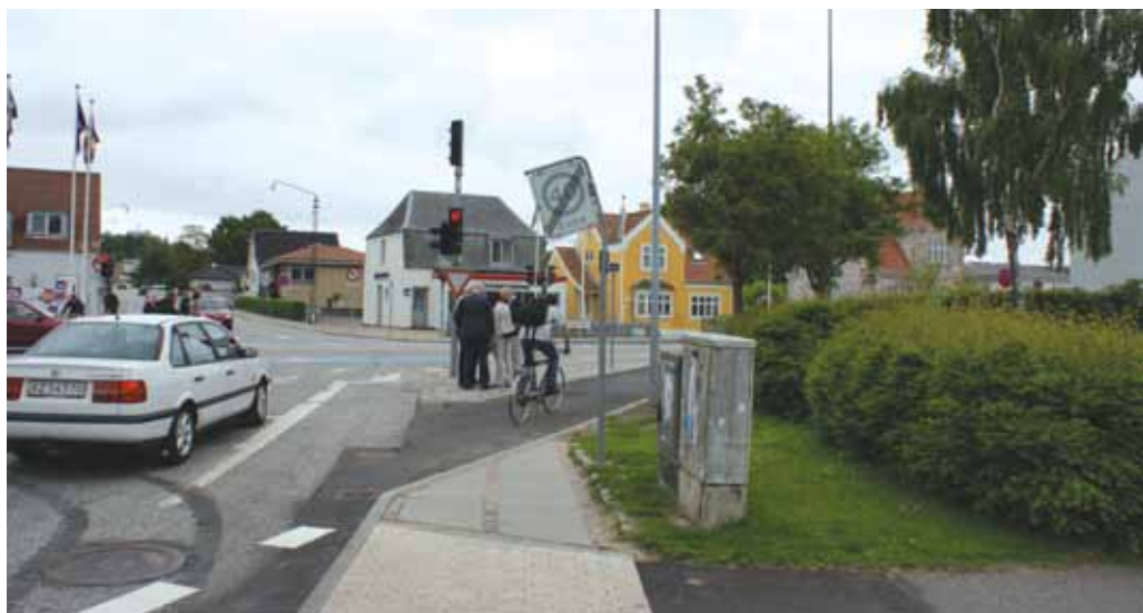
Shunt in Aalborg improves passability since cyclists needn't wait for the green signal before turning right.
