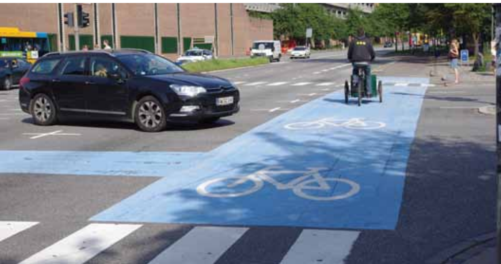
Internal road safety considerations in the City of Copenhagen tend toward using up to 2 blue cycle crossings per intersection, based on a concrete assessment of the individual situation. Tagensvej.
