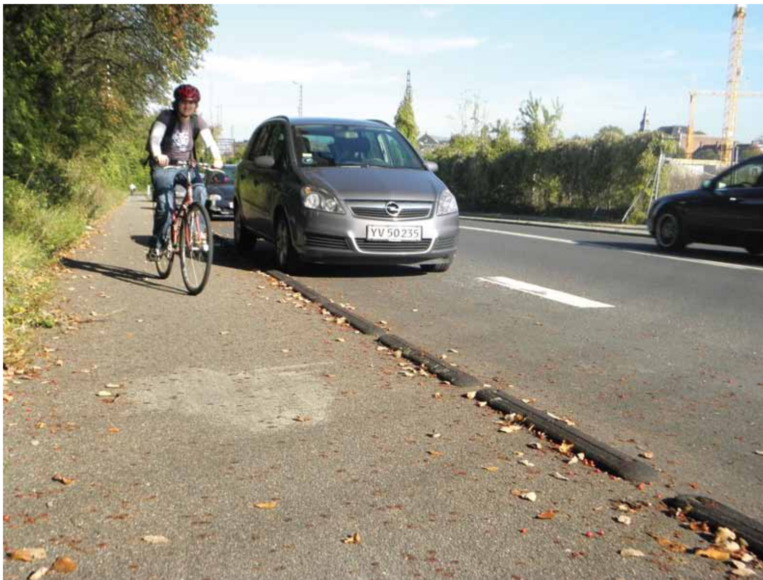
A cycle lane delineator like this one can work on roads with very few crossing pedestrians. It's cheaper and doesn't require drainage facilities.
